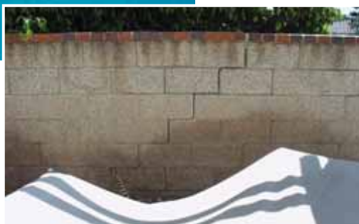
Side property line walls will crack usually 10 to 15 ft. from the slope.
