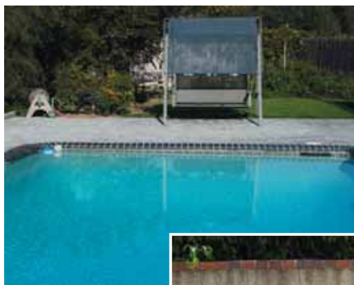
Pool rotates and becomes out of level. Note water line at tile on left slope side versus right side.
